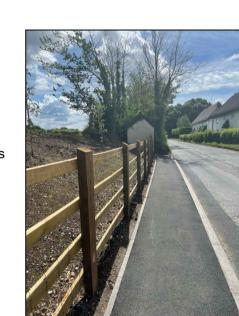
Existing Phase 1 footway to continue along Phase 2 in front of bus shelter providing a continuous footway link.
